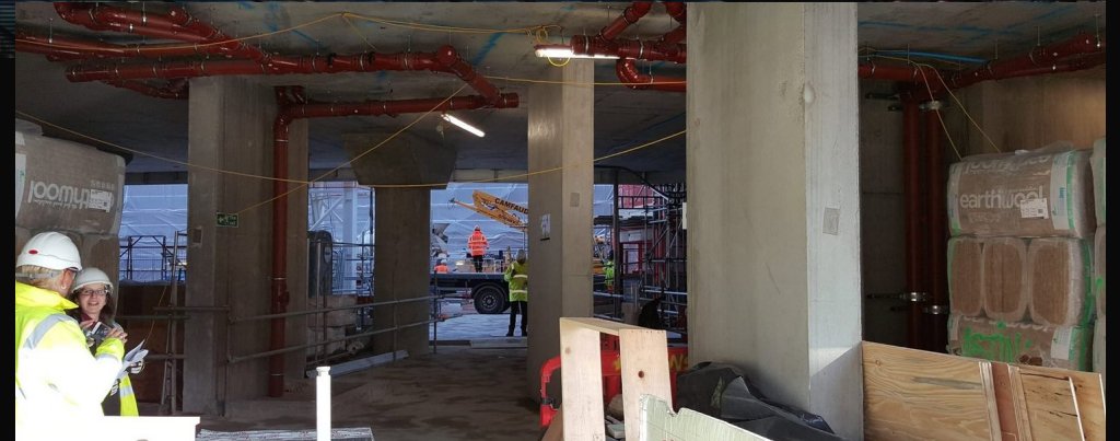
Pre construction site survey
