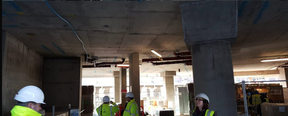
Structural frame and first-fix coordination
