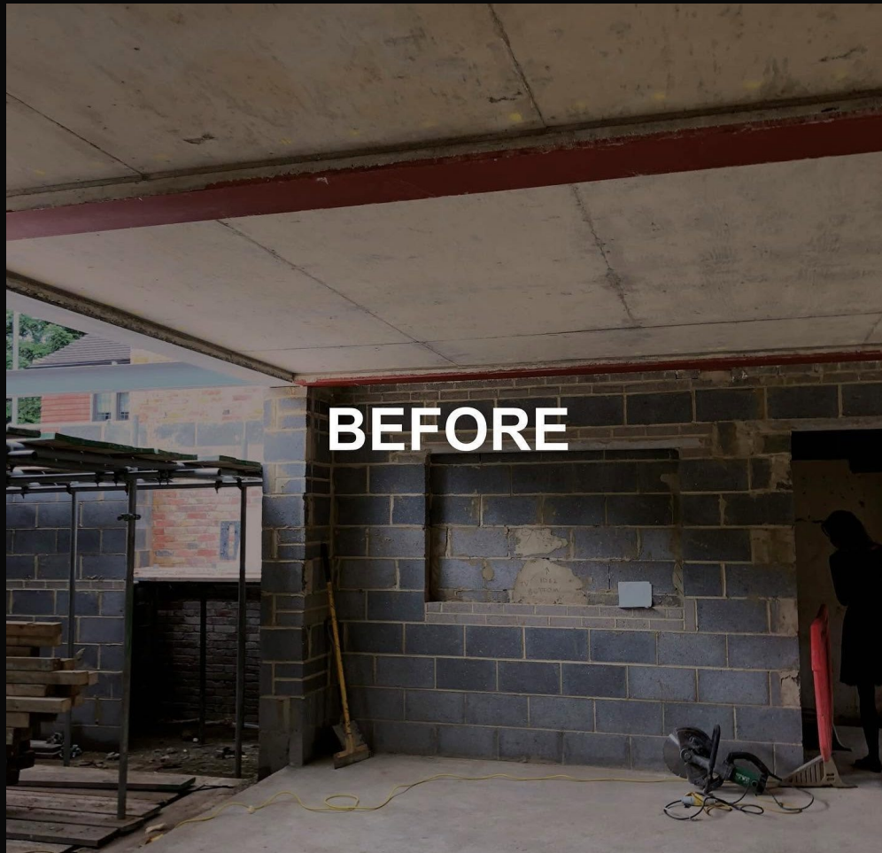
From structural shell to private entertainment suite.
